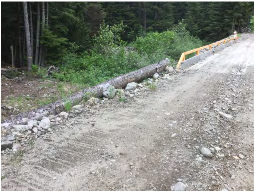
Small fender logs - typical all 4 corners
