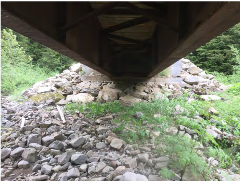
Left Bank Abutment when facing downstream
