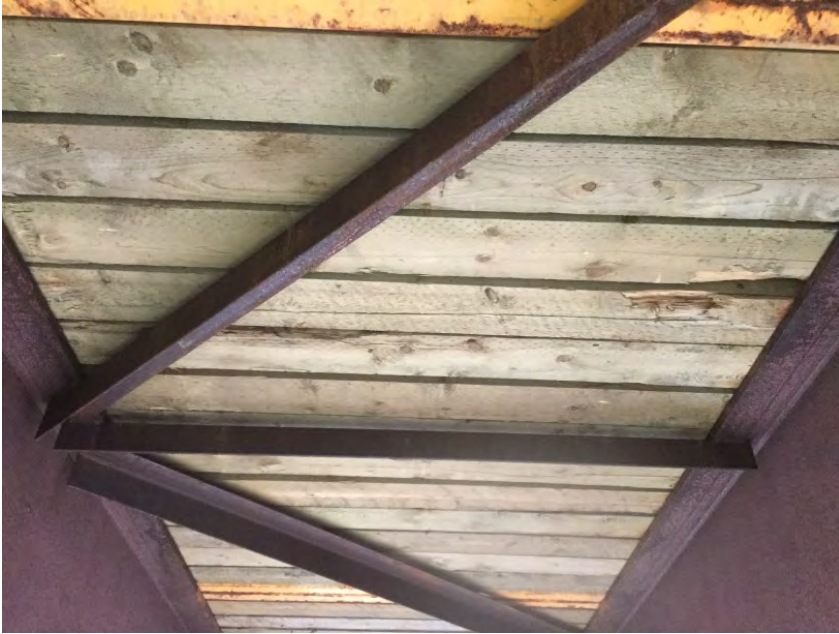
Deck from underneath
