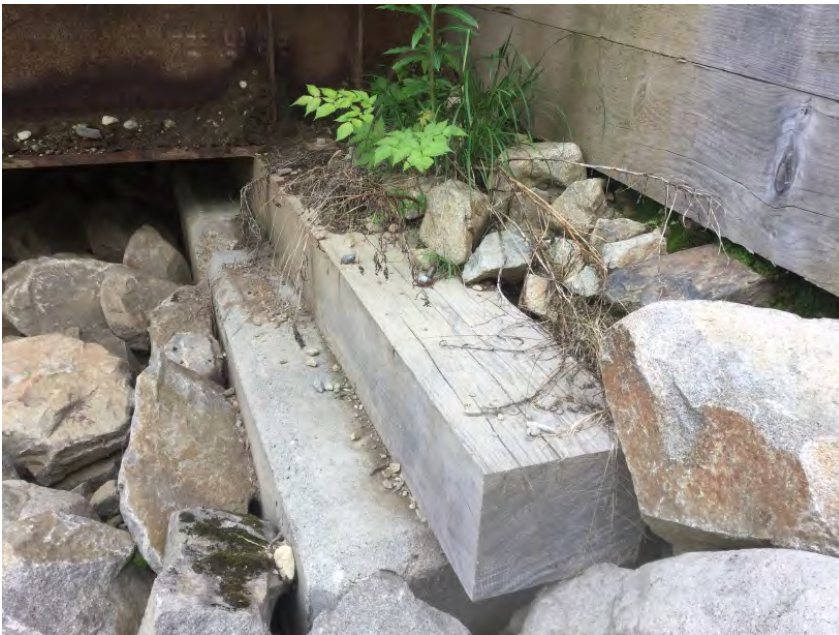
Sill - typical both sides
