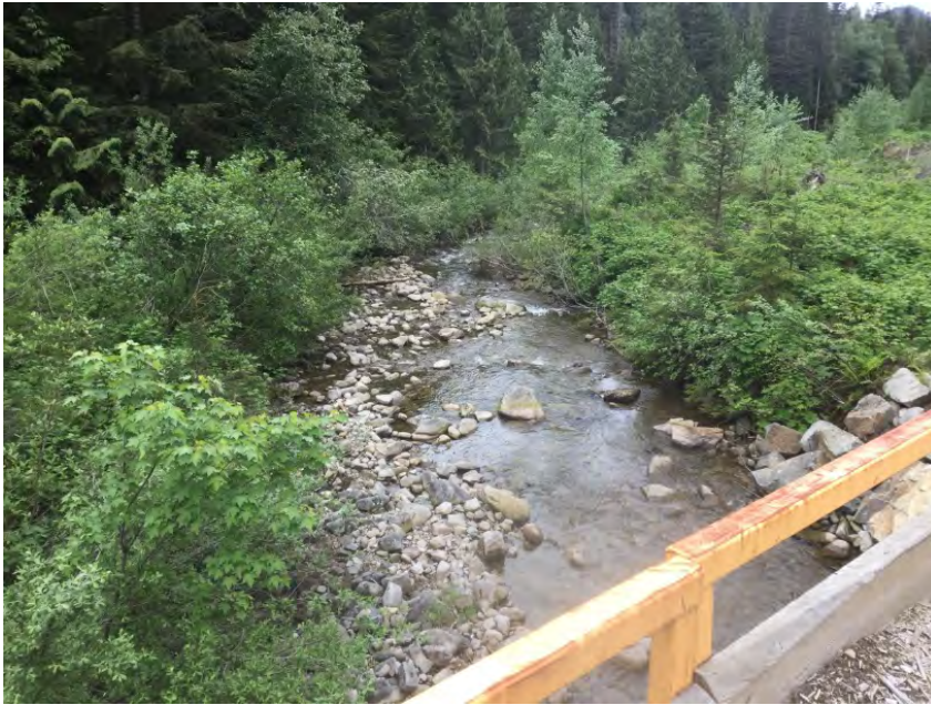
Looking downstream from deck
