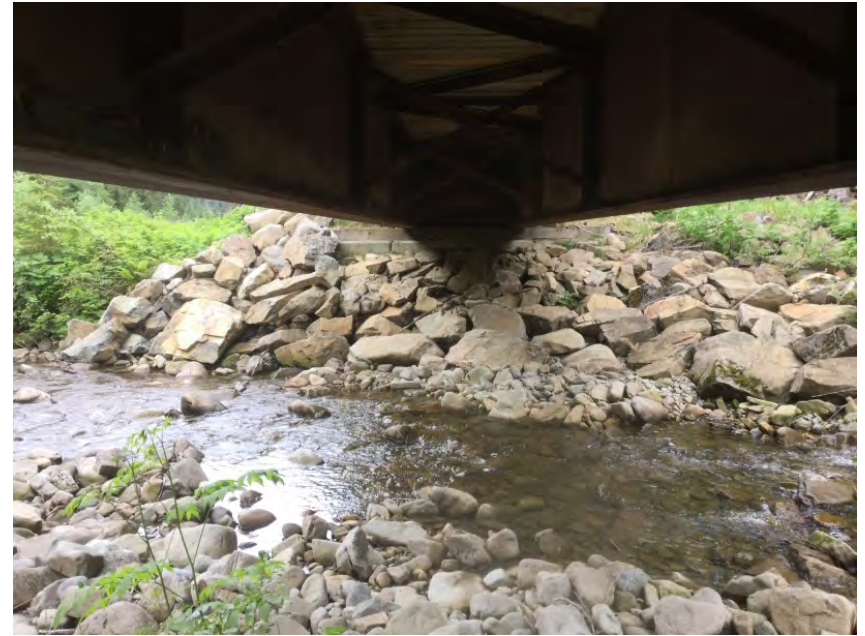
Right Bank Abutment when facing downstream
